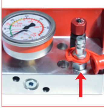
41. After positioning and hosing all the cylinders, proceed through the quick fit device through the control panel for charging all the cylinders. Make sure that the discharging valve is closed properly (15 Nm). 39DMCPVA control panel charging unit.
